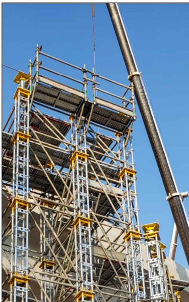
The versatility of the Ringlock Giantshore allows for standard working platform to be erected upon completion of the tower.
